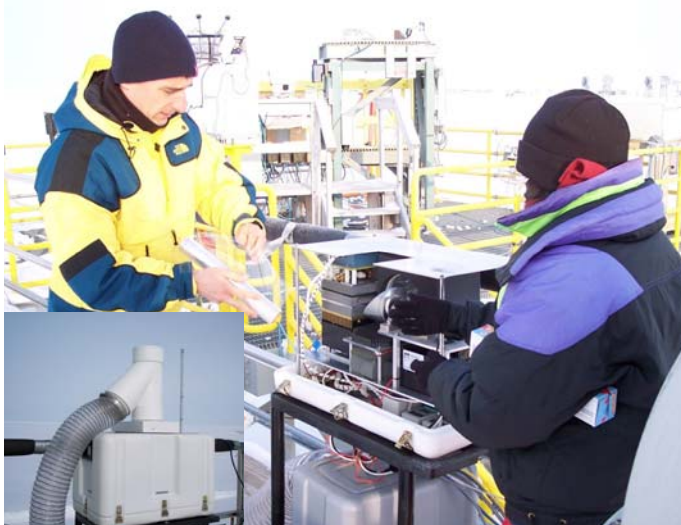
The 183 GHz radiometer, protected inside an insulated enclosure (inset), is installed on the roof of the primary instrument shelter at Barrow. To prevent snow from accumulating on the mylar window, a blower mounted beneath the radiometer directs air through a duct to a standard Y-shaped fitting mounted on top of the radiometer
